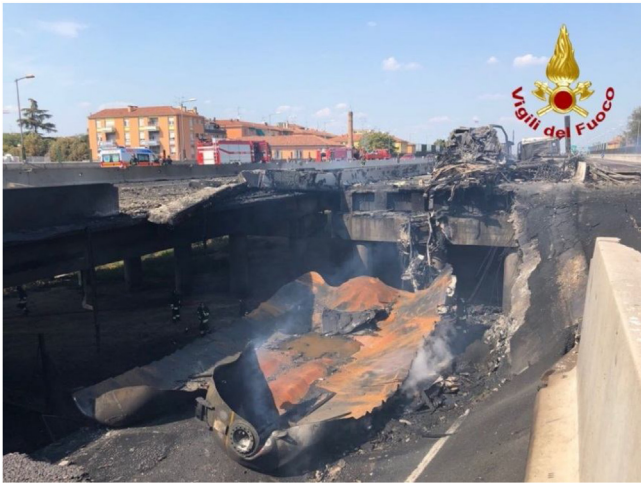
Fig. 1. Opened vessel and collapsed bridge after a tanker truck accident leading to a BLEVE on an elevated highway near Bologna, August 2018. Picture from the website of Italian firefighters (Vigilfuoco.tv, 2018).
