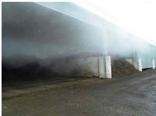
Figure 2: Picture of the fermentation area
